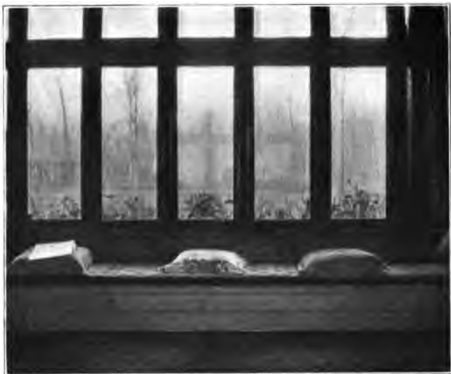
WINDOW BOX FROM INSIDE
